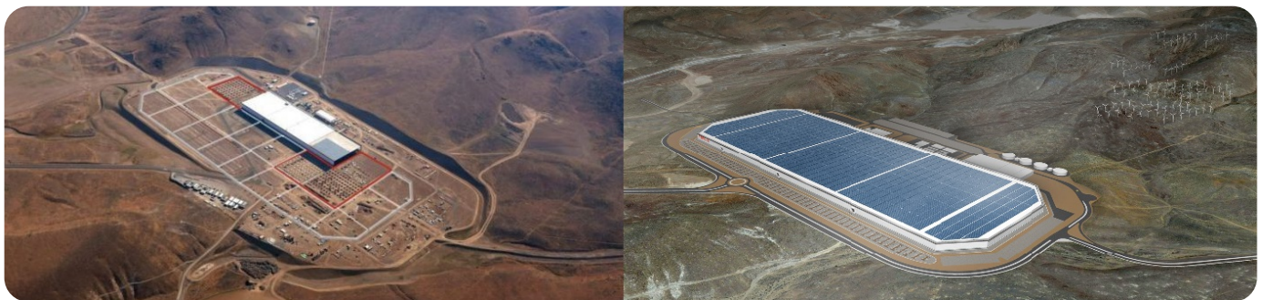
Tesla Gigafactory construction progress (sources: elektrek.co, tesla.com)
